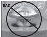
OVAL NECK OF BOLT NOT SEATED PROPERLY
