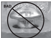
OVAL NECK OF BOLT NOT SEATED PROPERLY
