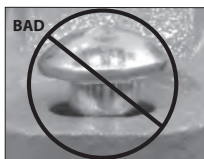
OVAL NECK OF BOLT NOT SEATED PROPERLY
