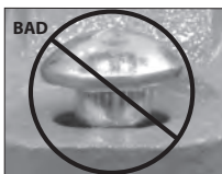
OVAL NECK OF BOLT NOT SEATED PROPERLY
