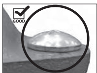
OVAL NECK OF BOLT SEATED PROPERLY
