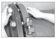
10. INSTALL REMAINING BOLTS/ NUTS: Insert a standard, full-shank diameter assembly bolt through each remaining hole in the Vic-Flange Adapter/ mating flange. Thread standard flange nuts finger-tight onto all bolts.
