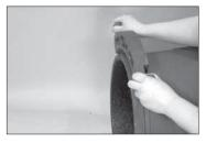
2. ADD FIRST SEGMENT: Place the first segment onto the pipe, making sure that the key engages in the groove properly. NOTE: On vertical pipe, the segments must be held in place until all segments are fastened together. For horizontal pipe, the segments can be balanced on top of the pipe, as shown above.
