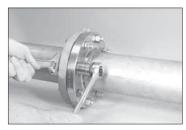
**9. TIGHTEN NUTS:** Tighten all nuts evenly in a crossing pattern, as with a standard flange assembly. Continue to tighten all nuts until the standard, flange-bolt torque recommendation is achieved.
