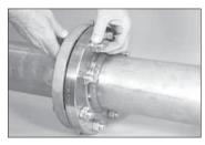
8. INSTALL REMAINING BOLTS/ NUTS: Insert a standard, full-shank diameter assembly bolt through each remaining hole in the Vic-Flange Adapter and the mating flange. Thread a nut onto each bolt until they are finger-tight.
