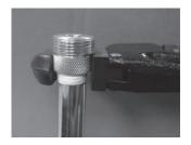
First step: Wrap several layers of pipe sealing tape over the threads of the steel pipe. Install the threaded end of dielectric union body to the steel pipe. Turn the union clockwise and tighten with a pipe wrench.
