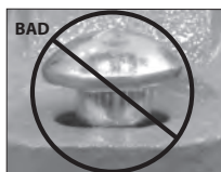
OVAL NECK OF BOLT NOT SEATED PROPERLY
