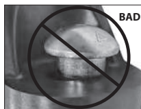
OVAL NECK OF BOLT NOT SEATED PROPERLY
