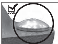
OVAL NECK OF BOLT SEATED PROPERLY
