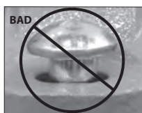
OVAL NECK OF BOLT NOT SEATED PROPERLY
