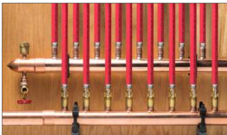
Radiant Manifolds Allow for fine-tuning of supplied water volume to radiators or tubing loops (not shown in illustration)
