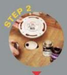
Put toilet flange onto drain and make solvent weld connection.
