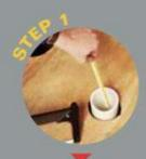
Cut pipe to fit inside of toilet flange.
