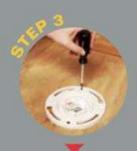
Secure toilet flange to floor with fasteners.
