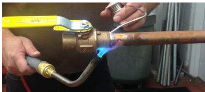
Figure 2 – Heat valve cup area and apply solder
