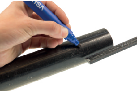
FIGURE 8: MARKING INSERTION DEPTH
