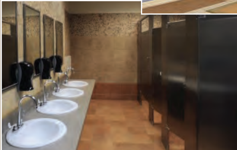
Restroom Partition Hardware
