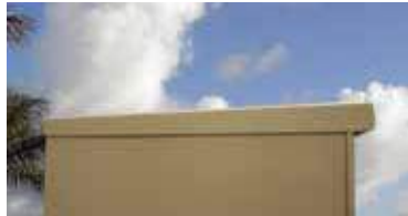
Sloped top for moisture runoff
