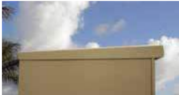
Sloped top for moisture runoff
